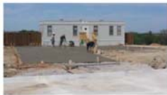
Work in progress on Serene Homes information Center
