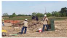
Workers pulling power lines into power box
