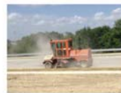
Cleaning of roads in phase one
