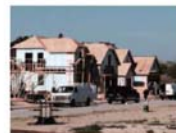
Exterior of Model Homes 50% complete
