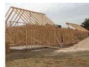
Roofing of Model Homes
