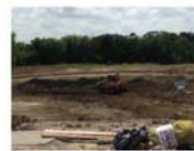
Laying clay in Storm Water Management Pond
